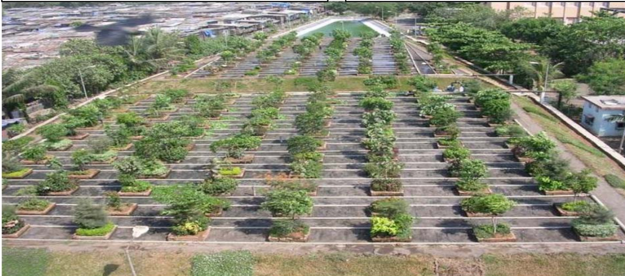
3000 KLD plant at BMC (Worli), Mumbai
