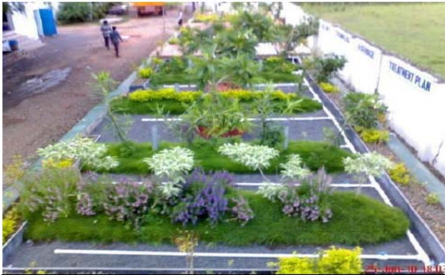
25 KLD plant at Godrej, Pondicherry
