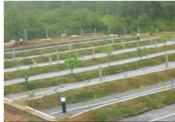
75 KLD plant at FRLHT Hospital, Bengaluru
